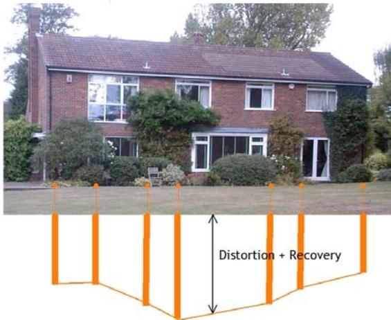
Both flank walls show downward slopes towards the rear corners of the house of 40 – 46mm possibly implicating the surrounding trees. The maximum distortion has the Wisteria as a focal point, one-third the way along the rear house wall.
